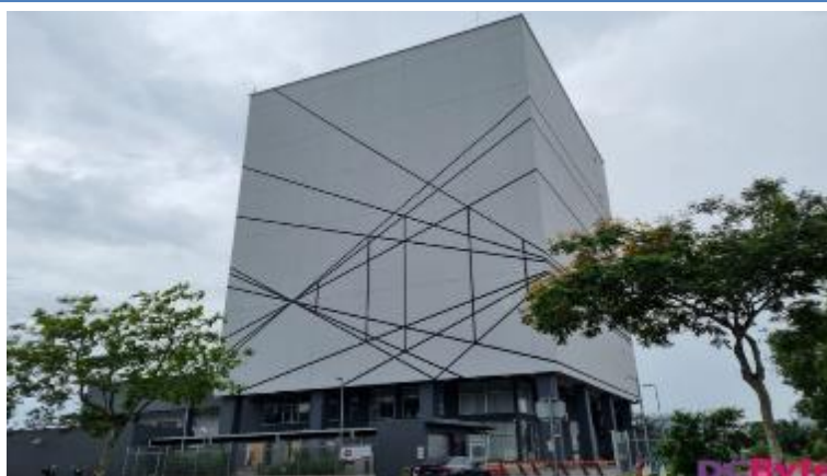
Figure 11: AIMS' first data centre in Cyberjaya
